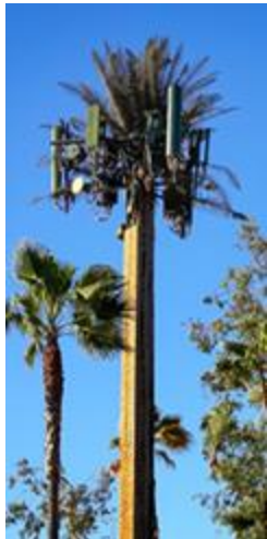
Telecom site over a fake palm tree
