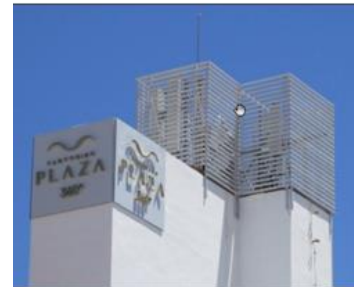
An example of cladding screening
