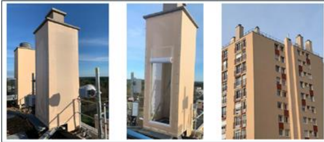
A chimney based on mesh material (France)
